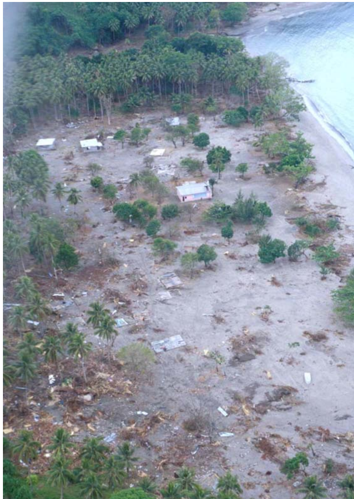
Figure 1. The village of Baie Martelli after the tsunami. Only concrete buildings remain standing, and those are too badly damaged to remain inhabited. The large structure in the center of town is the village church. Water surged over the top of the church (4.25 m above ground surface), crushing its corrugated metal roof.
